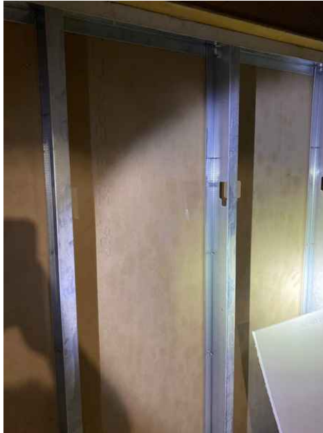
Basement Wall Framing/Steel Studs
