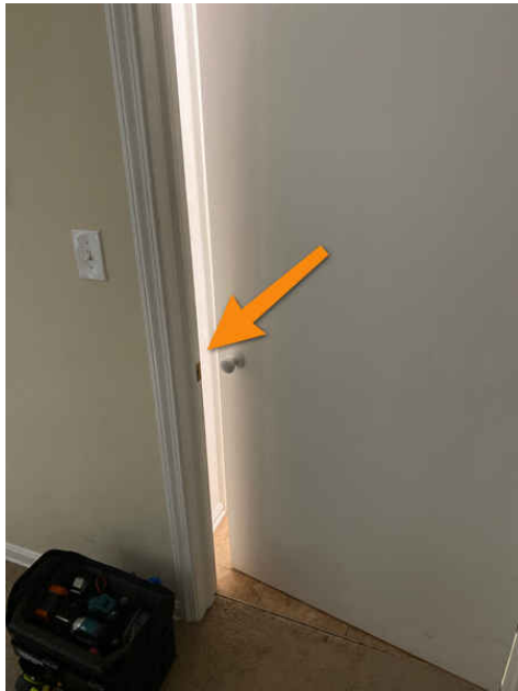
Entryway Door Doesn't Latch
