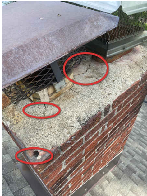
Cracked Crown
