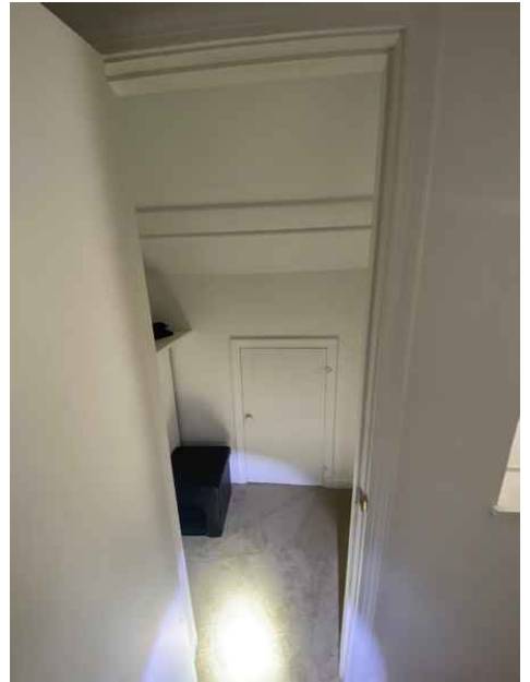
2nd Floor storage closet
