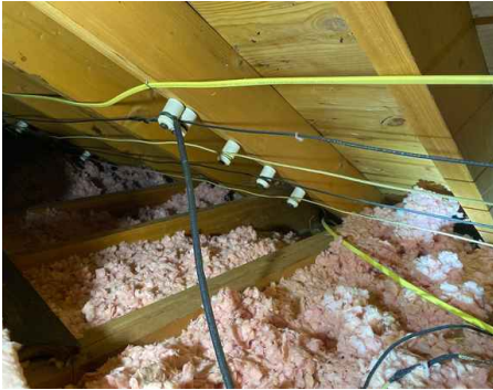
Active Knob and Tube/Attic
