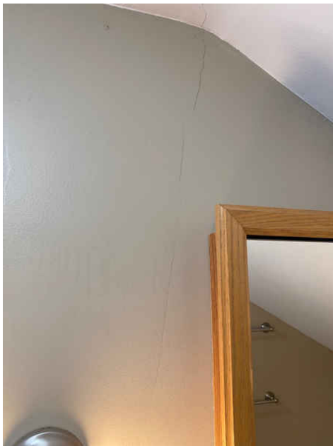
Wall Cracks
