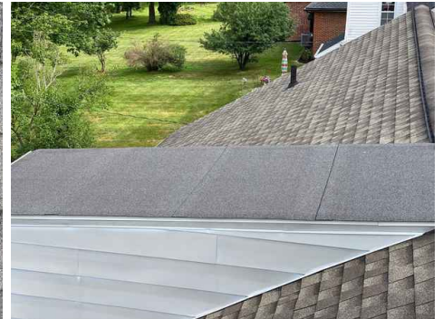
Dormer Shed/Flat Roof with Rolled roofing
