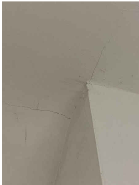
Ceiling Cracks
