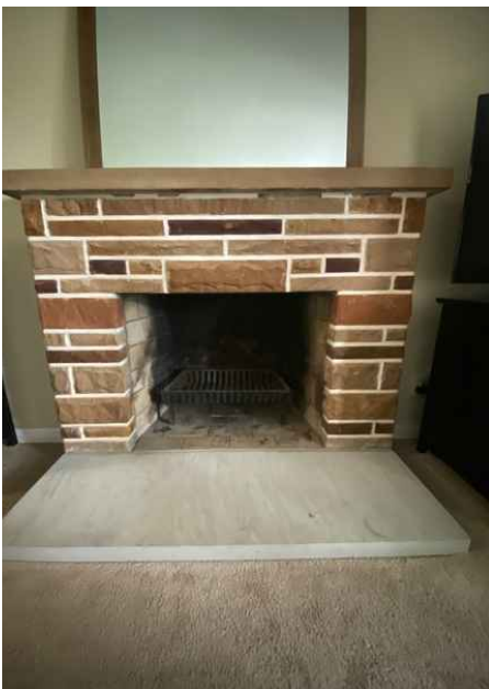
1st Floor Front Room Fireplace
