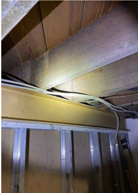
Steel I Joist Beam
