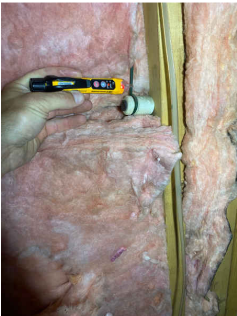
Active Knob and Tube wiring/insulation Active Knob and Tube wiring/insulation
