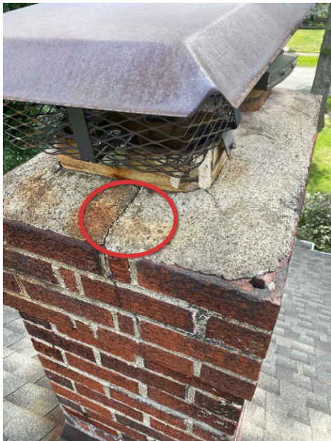
Cracked Crown
