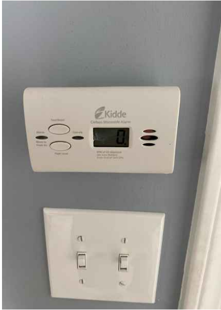
1st Floor Bedroom
