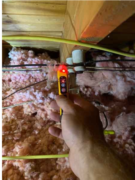
Active Knob and Tube/Attic
